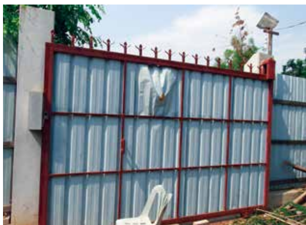
Damaged compound, Yesagyo. Photo: Rachel Fleming
